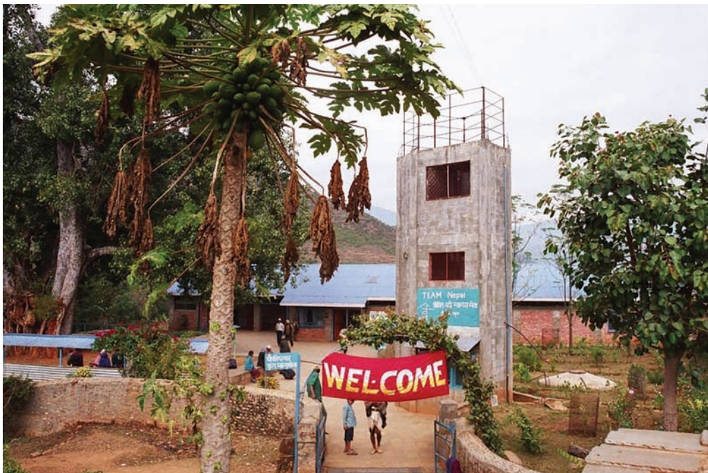
Rukum Hospital, a small rural hospital in mid-western region of Nepal.
